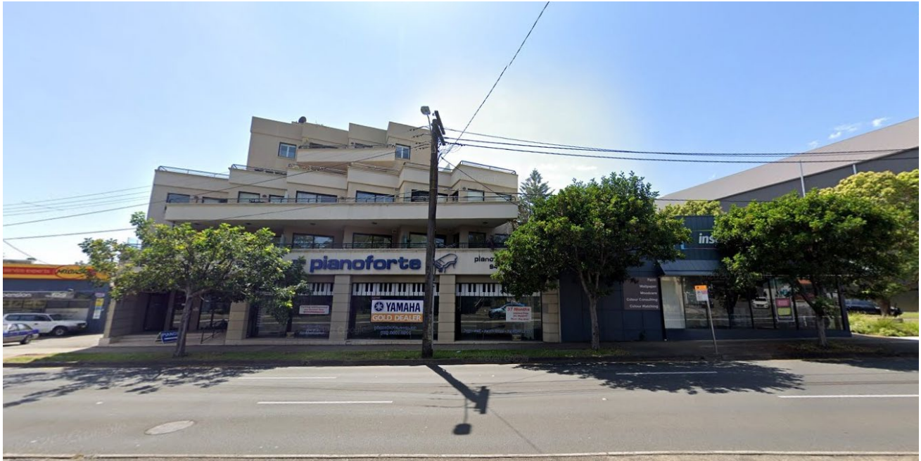
Figure 3 View of the site front Pacific Highway
